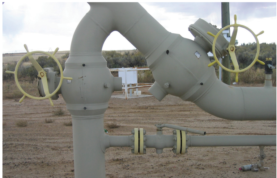
While double block and bleed valves are most often used in the oil and gas industry, they also are employed in other industries, particularly when piping isolation is essential and leakage must not occur.
