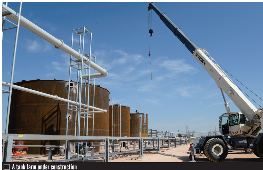
□ A tank farm under construction
