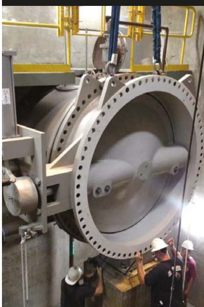
Figure 1. Installation of 90-inch butterfly valve
