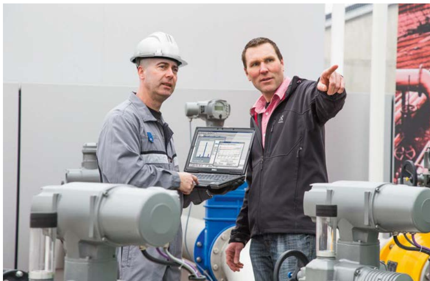
□ Commissioning is often performed by the company that installs the equipment.
