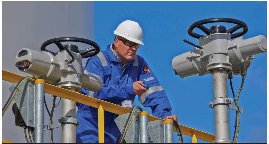
□ Manufacturer's technician accessing the electric actuator data logger to diagnose a performance issue.
