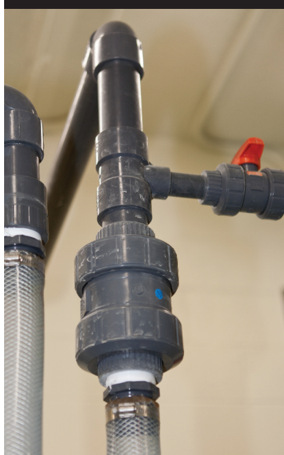
□ Figure 4. A ball check valve installed vertically
