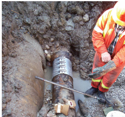
□ A repair worker locates the source of a water main break.
